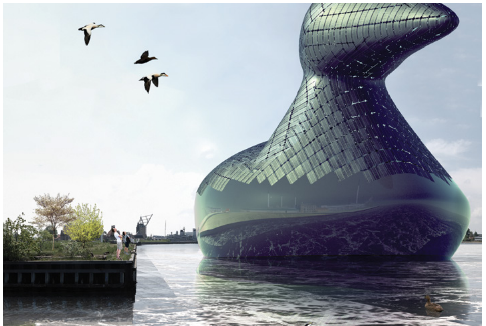
Energy Duck: A submission to the 2014 Land Art Generator Initiative design competition for Copenhagen Team: Hareth Pochee, Adam Khan, Louis Leger, Patrick Fryer Energy Technologies: Photovoltaic panels, hydraulic turbines (Kaplan, Francis, or similar 100–500 kW capacity) Annual Capacity: 400 MWh
